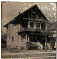
A No. A-241 IDEAL Boiler and 461 sq. ft. of 38-in. AMERICAN Radiators, costing owner $215, were used to heat this cottage. At these prices the goods can be bought of any reputable, competent fitter. This did not include cost of labor, pipe, valves, freight, etc., which are extra and vary according to climatic and other conditions.
